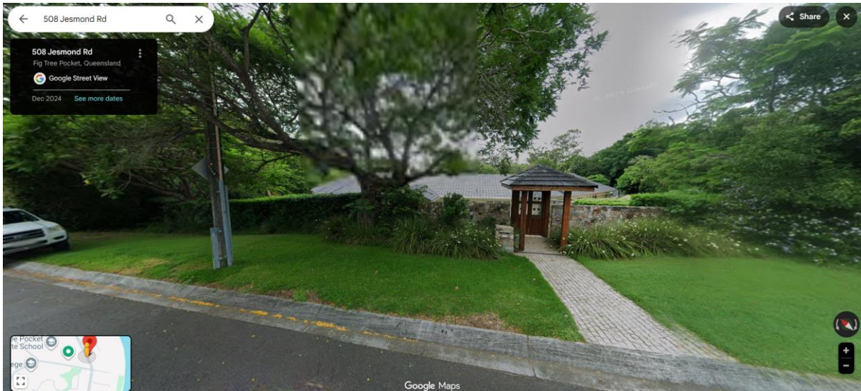
Figure 2-5 Site viewed from Jesmond Road
