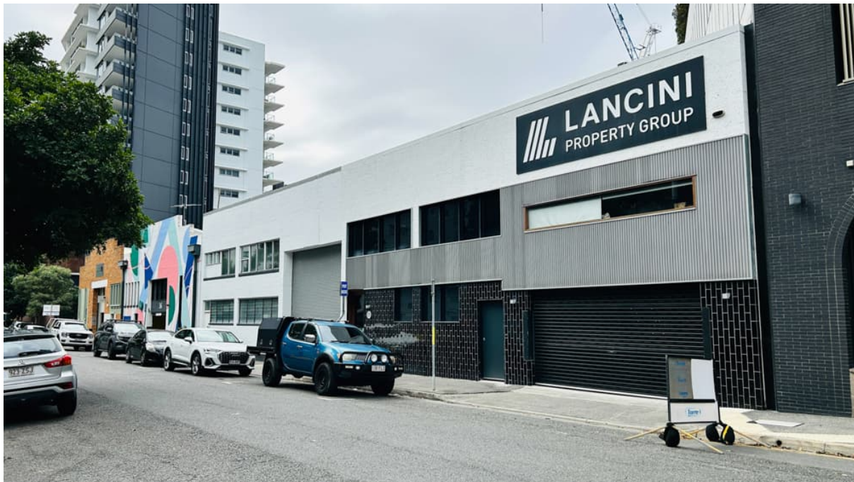
Figure 3 - View of Subject Site along Wyatt Street
