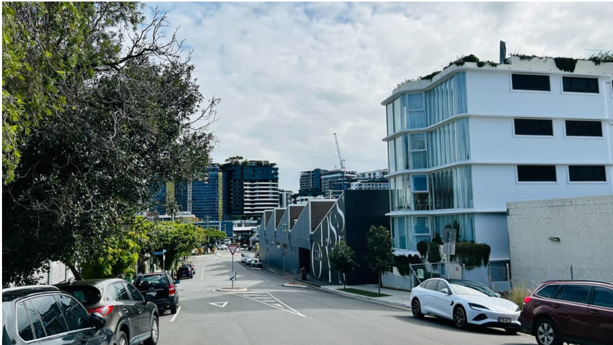
Figure 9 - View northwest to Subject Site from Chermide Street
