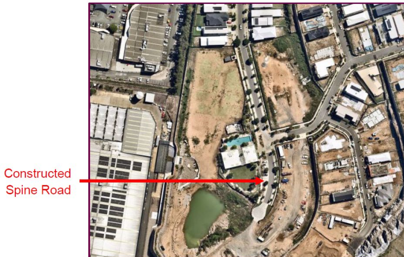
Figure 2 – Constructed Spine Road (servicing Stages 101, 102 and 105)
