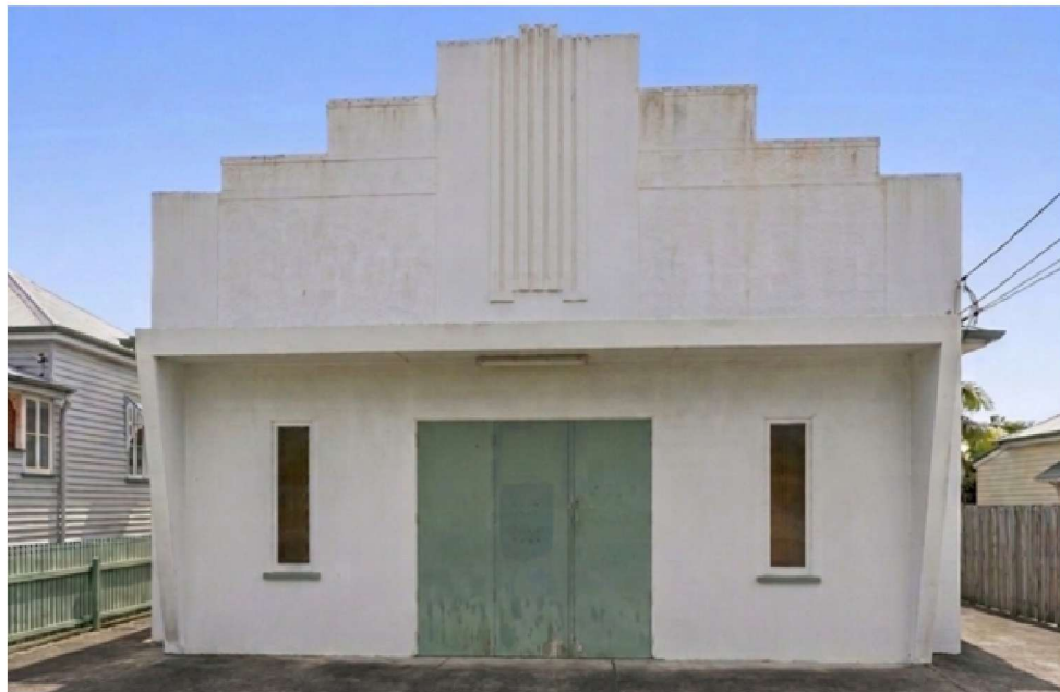
Existing Front View
